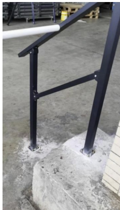
Photo 3 Connection between handrail and column in the test
