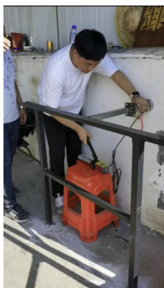
Photo 5 Load test loading
