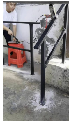
Photo 4 Load test loading
